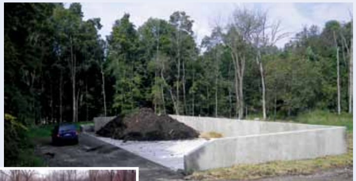
AFTER: This completed storage facility in Putnam County now effectively contains manure while directing runoff to a vegetated treatment area. A local plant nursery owner in need of compost now hauls out the material for free. The area adjacent to the facility was seeded and now serves as a buffer between the facility and a watercourse. Clean storm water from an indoor riding arena roof upslope from the facility is now diverted around the area with the installation of a drip trench and underground outlet.
