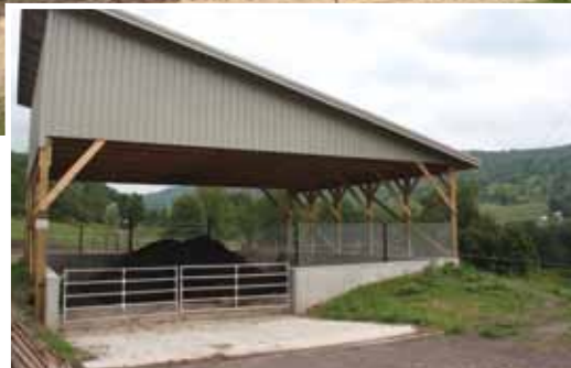
New facilities allow for manure to be collected, stored, and spread in accordance with a Nutrient Management Plan. The Whole Farm Plan incorporates water quality practices that prevent nutrient-laden run-off from entering nearby streams.
