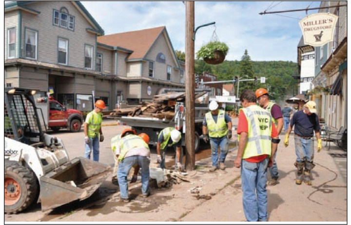
AT WORK: DEP crews in Margaretville provide clean-up assistance on August 31.
