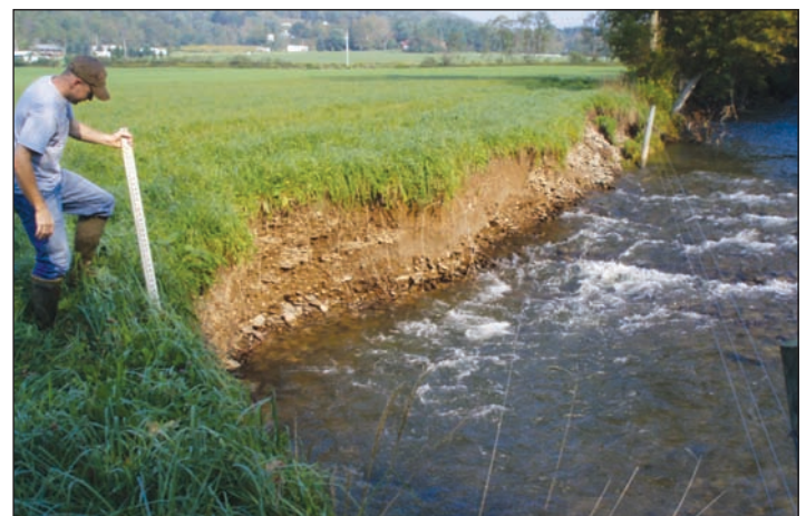
Streambank stabilization will prevent further erosion but won't remedy lost pasture or replace rental acreage enrolled in federal programs.
