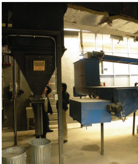
Figure 3. A multicyclone filters particulates at Springfield High School's wood chip system.
