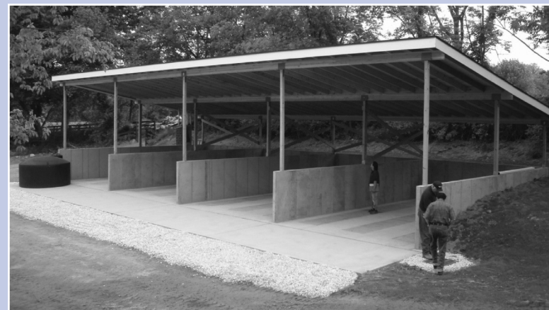
Front view of forced-air composting facility: Each of the four bays of this facility are 15.5 feet wide, 5 feet high, 30 feet deep and can hold approximately 83 linear cubic yards of material. Each bay was also constructed with 3 aeration boxes (wooden slats shown in the photo above) to allow air to circulate through the material resulting in decreased composting time. Compost cycle time would be decreased to approximately 30 days and cured in a separate area for 60 days.
